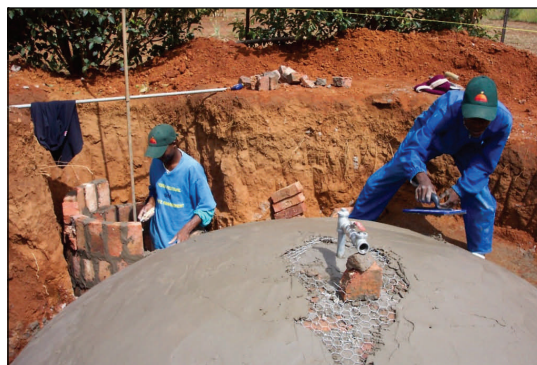
Biogas plant under construction in Africa
