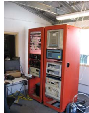
Continuous emission monitors
