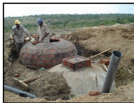
Construction of a fixed dome biodigester
