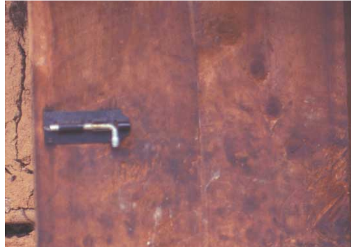
Enlarged windows let air into the home
